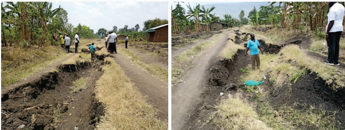
Roads leading to a primary school in Nalugugu parish relentlessly destroyed as a result of floods disaster
